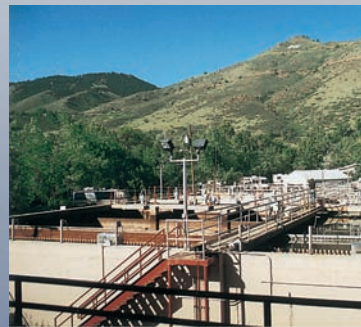
THE GOLDEN WATER TREATMENT PLANT, COLORADO—THIS FACILITY IN SCENIC GOLDEN HANDLES SEVERAL MILLION GALLONS MORE PER DAY WITHOUT ANY INCREASE IN BASIN SIZE OR LAND AREA, THANKS TO MRI PLATE SETTLERS.
