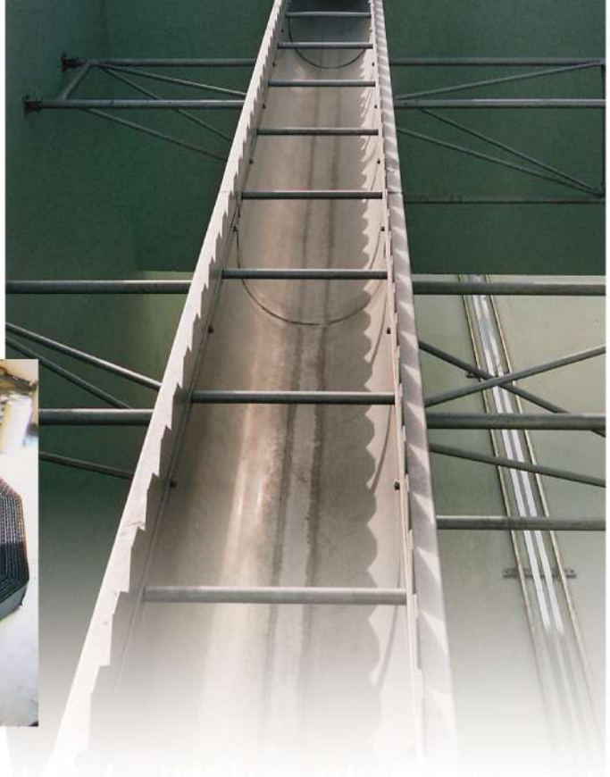
Pictured above: ARAMCO Water Treatment Facility, Saudi Arabia—Includes MRI round bottom stainless steel collection troughs and stainless steel supports.
