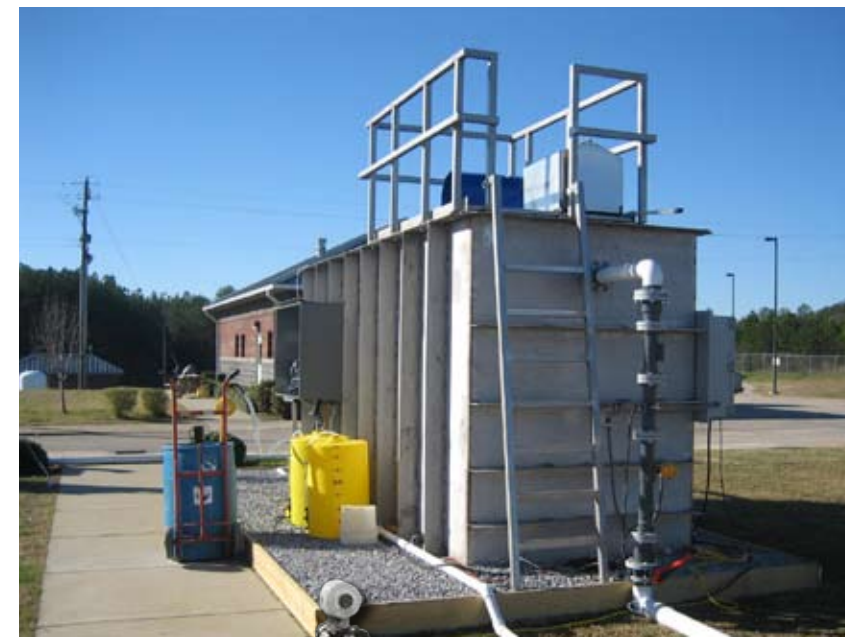
LARGE MRI PILOT SYSTEMS ARE USED TO ESTABLISH PROCESS PROTOCOLS, WHICH ONCE OPTIMIZED, ARE SCALED AND APPLIED TO THE FULL WATER TREATMENT PLANT.
