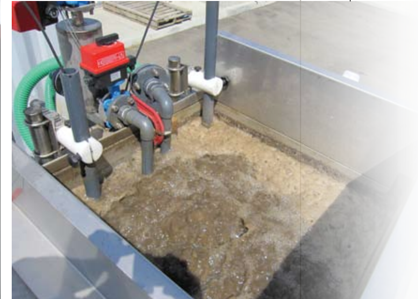
LEFT - INSIDE OF CONTROL PANEL CENTER - MEMBRANE FILTER TANK SHOWS AIR CONTROLS AND INSTRUMENTS. RIGHT - MEMBRANE FILTER TANK IN OPERATION CONTAINS MIXED LIQUOR SUSPENDED SOLIDS UP TO 12,000 PPM.
