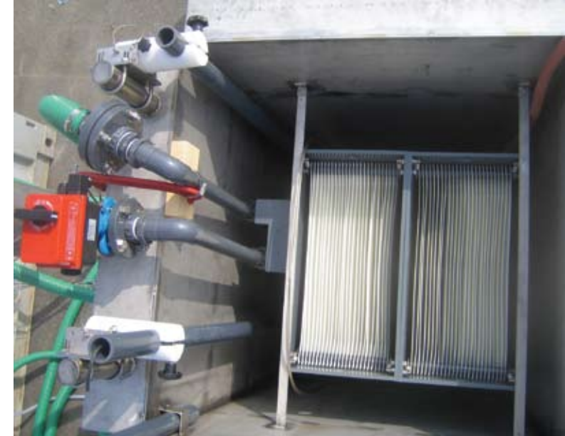
LEFT - INSIDE OF CONTROL PANEL CENTER - MEMBRANE FILTER TANK SHOWS AIR CONTROLS AND INSTRUMENTS. RIGHT - MEMBRANE FILTER TANK IN OPERATION CONTAINS MIXED LIQUOR SUSPENDED SOLIDS UP TO 12,000 PPM.
