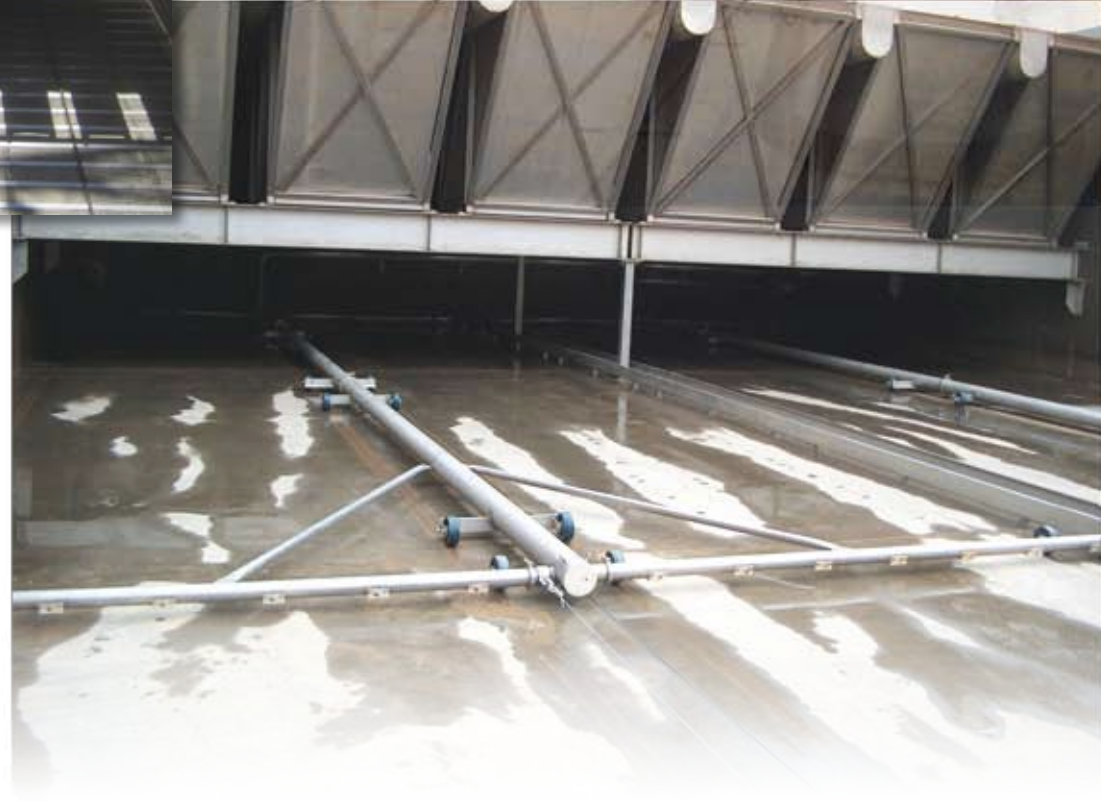
THE WATER TREATMENT PLANT IN PIEDMONT, AL WAS COMPLETELY REFURBISHED WITH THE MRI RETRO CABLE-VAC. (TOP)
