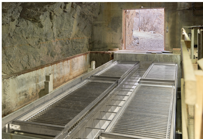
MRI Inclined Plate Settlers in No Name Cave are custom designed, featuring larger-diameter openings on the patented top tube distribution surface. These openings handle higher loading rates to accommodate for the limited available space.
