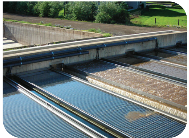
Agitation shown. Water level usually lowered to avoid carryover.
