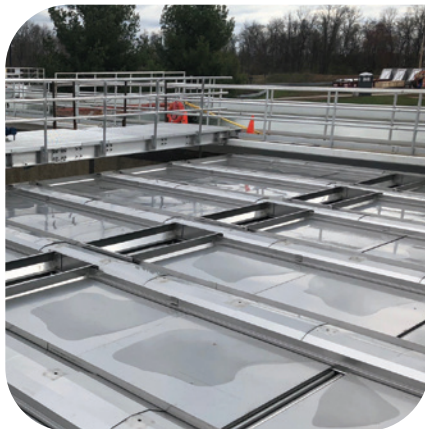
Active plate pack with left side exposed and prone to algae growth and right side covered.
