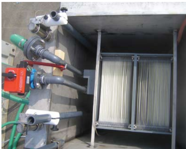
LEFT - INSIDE OF CONTROL PANEL CENTER - MEMBRANE FILTER TANK SHOWS AIR CONTROLS AND INSTRUMENTS. RIGHT - MEMBRANE FILTER TANK IN OPERATION CONTAINS MIXED LIQUOR SUSPENDED SOLIDS UP TO 12,000 PPM.
