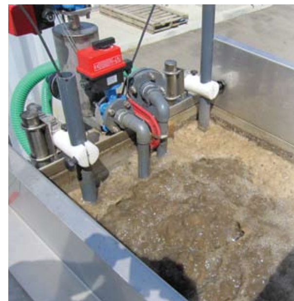
LEFT - INSIDE OF CONTROL PANEL CENTER - MEMBRANE FILTER TANK SHOWS AIR CONTROLS AND INSTRUMENTS. RIGHT - MEMBRANE FILTER TANK IN OPERATION CONTAINS MIXED LIQUOR SUSPENDED SOLIDS UP TO 12,000 PPM.
